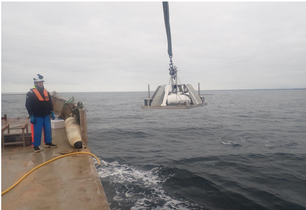
Figure 8 : Benne Day (cliché TBM)
